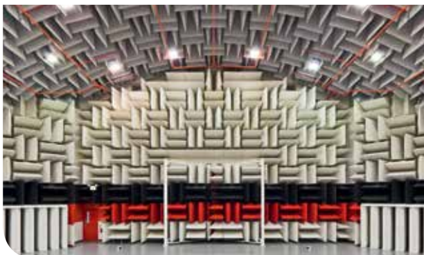
Hemi-anechoic room highlighting IAC's chosen lighting system alongside the client's preferred fire suppression system
