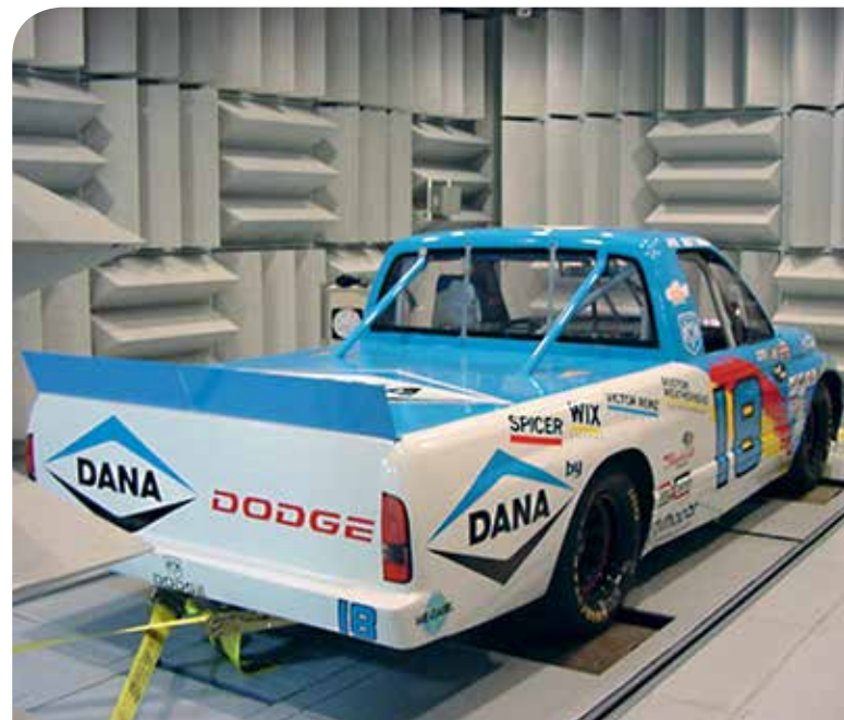
Hemi-anechoic chamber for Dana Trucks, USA
